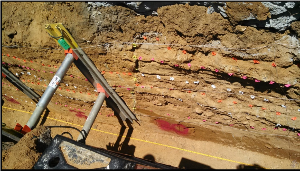
Figure 12 – At GDC Site 3, locality S2-11, view looking easterly at faulted Pleistocene alluvial fan deposits, yellow flag indicates fault to right of shoring near the center of the photo. Gray zone at the top of the photo is concrete. Bedding gently dipping to the south (right), with steepness increasing to the south. Of the 7 faults CGS observed, most faults indicated a difference in unit thickness across fault. The southernmost fault did not have any correlative units across the fault.
